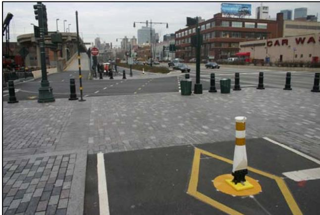
The styles and specifications of the bollards differ along the Hudson River Greenway and makes for an excellent study area. The use of bollards as both a design and safety feature and can be seen throughout the length of the greenway. Flexible plastic bollards are used on the inside of the path, while permanent steel bollards have been installed at path entrances and along the highway median.
